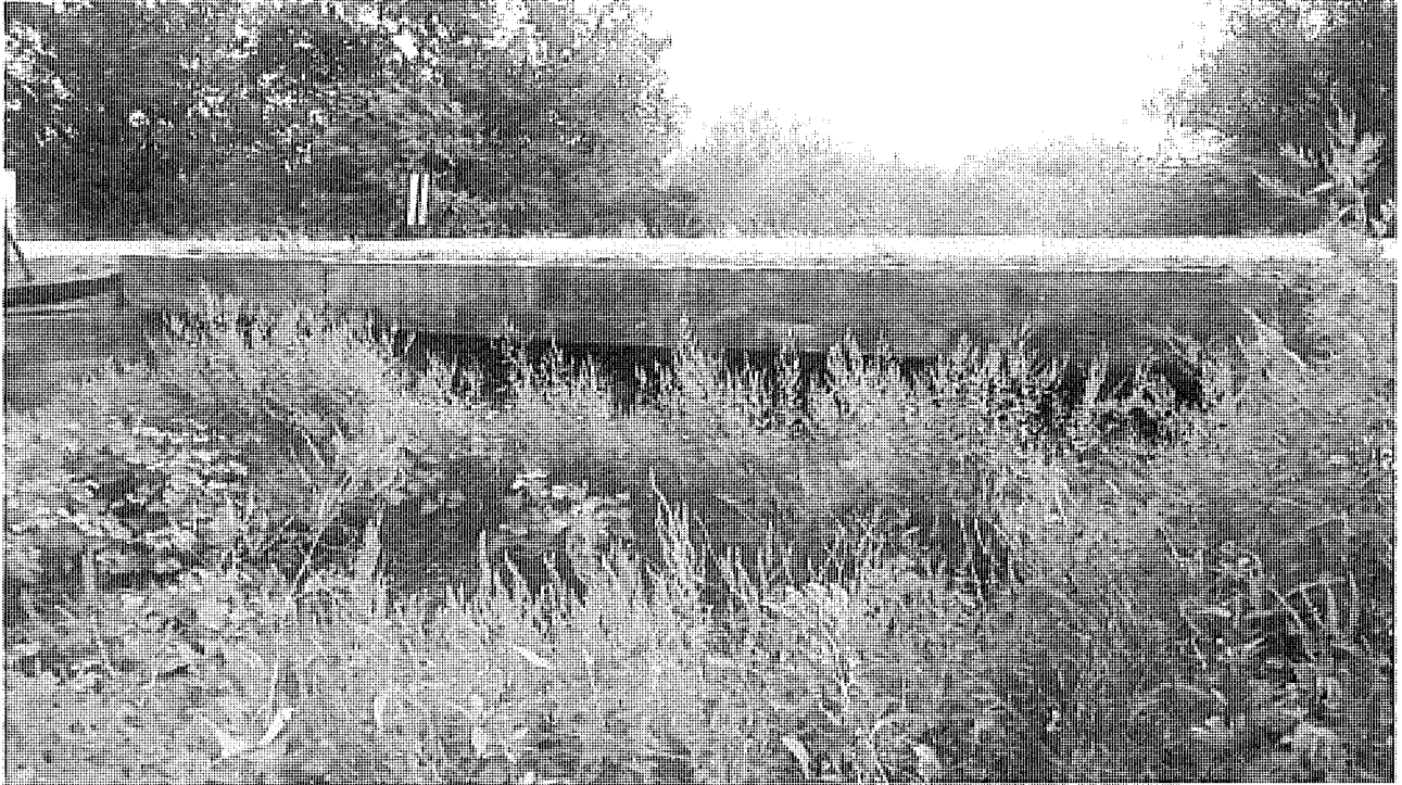
Figure 2: Culvert at Unnamed tributary of Elm Creek
